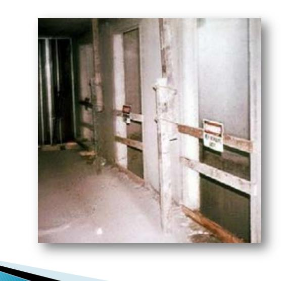
Unguarded floor openings must be guarded with a standard guardrail, or covered with a fixed cover.
