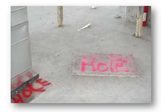
This includes any opening measuring 12 inches or more in its least dimension in a floor, platform, pavement, or yard, through which persons may fall.
